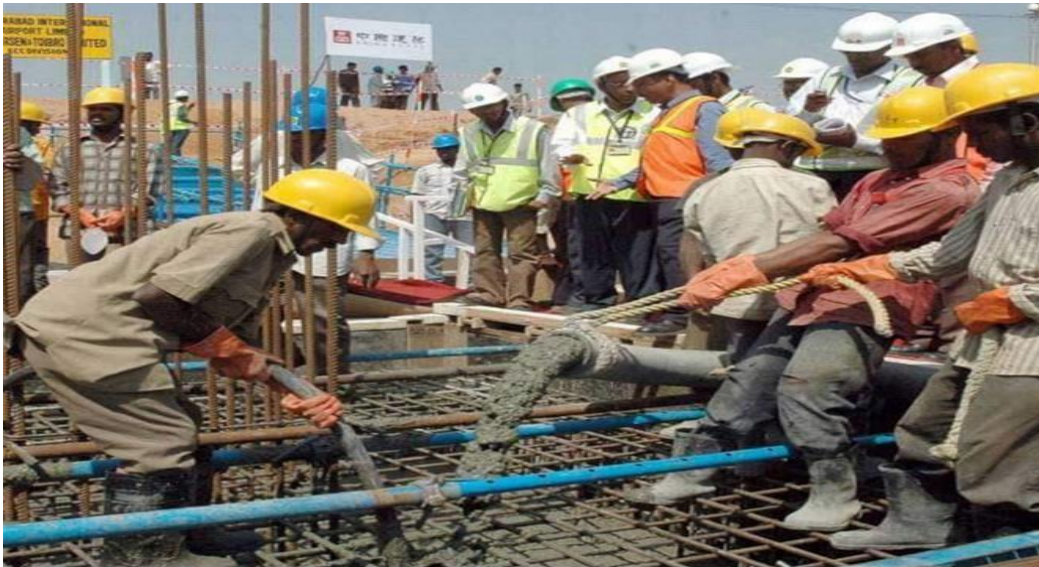
Fig.3: Placing and compacting concrete
